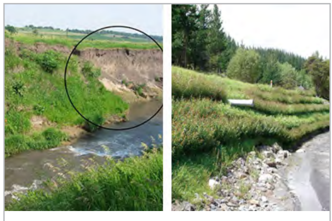
Left: Severe bank erosion; Right: A bio-based bank stabilization structure.
