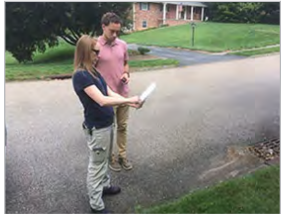
TNWRRC Intern Sean Ryan and Lori Saal, the Farragut Stormwater Manager, are reviewing the attributes needed to describe the stormwater grates.
