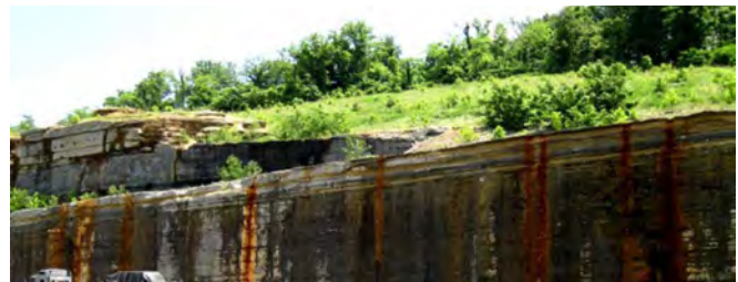
Road cut in Williamson County, Tennessee with signs of acid rock
