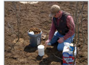
Wesley Wright, UT BESS, installs a sensor to capture flow rates in the Harrell Road rain garden.
