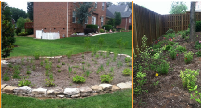
Newly installed rain garden at Cedar Crossing subdivision
