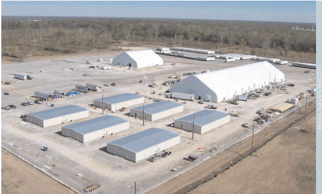
The FEMA morgue in Carville, Louisiana, was built in the aftermath of Hurricane Katrina. The facility, which cost $17 million to build and equip, operated for 10 weeks during the identifications of the hurricane's victims.
