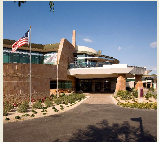
Photo courtesy of Douglas Fredrikson Architects, Inc.
